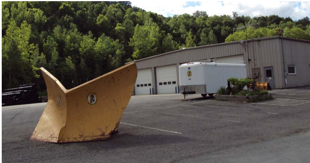
Photo 20 The Rensselaer County Highway Substation on Sand Bank Road
