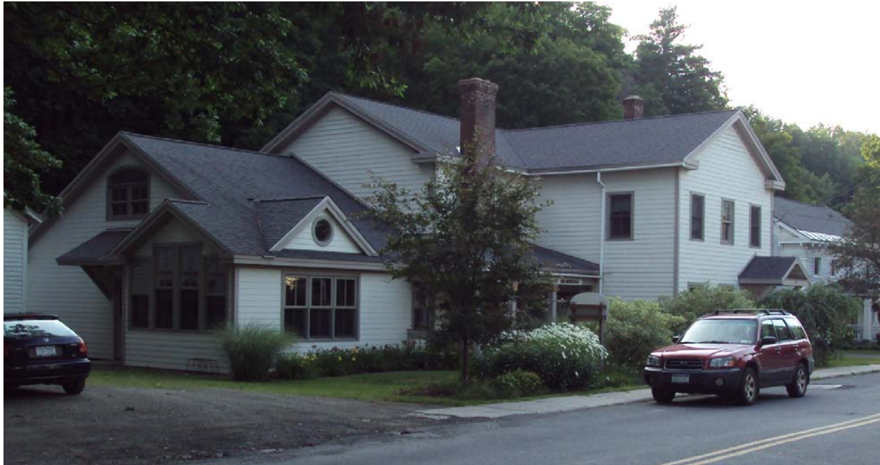
Photo 31 The Berlin Free Town Library is an example of a residence that has been repurposed as a public building.
