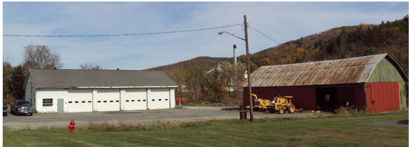
Photo 19 The Town of Berlin Highway Garage.
